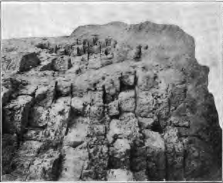
CRUMBLING WALLS OF REI
